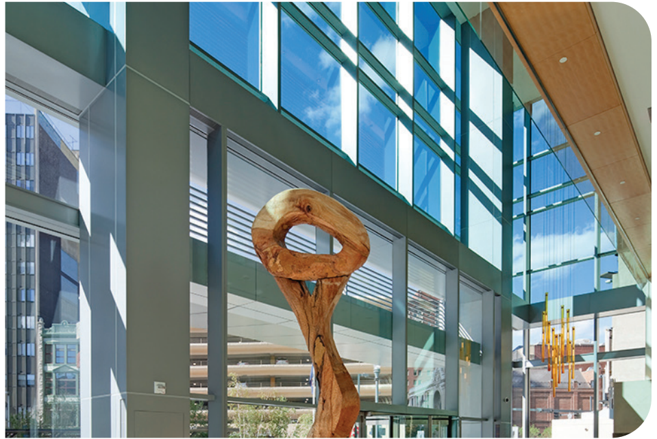
Three PNC Plaza is LEED-certified at the Gold level. The use of Solarban ® 60/clear and Solarban ® 60/ Starphire Ultra-Clear ® glasses provides the interior lobby with high levels of natural daylight while mitigating the effects of solar heat gain.
